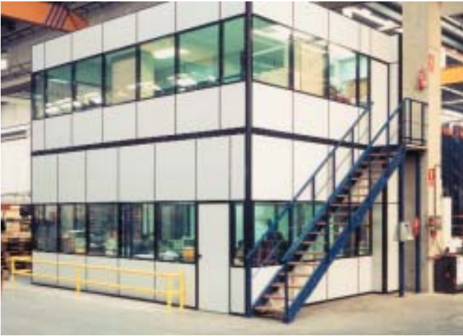
Mezzanine with offices for the control and management area installed in a factory.
